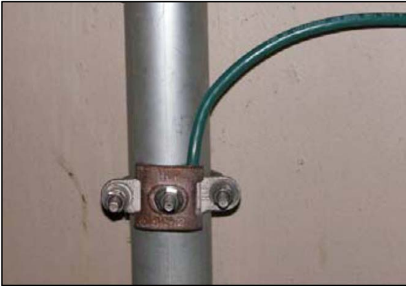
Figure 5. Example of a mechanical connector
