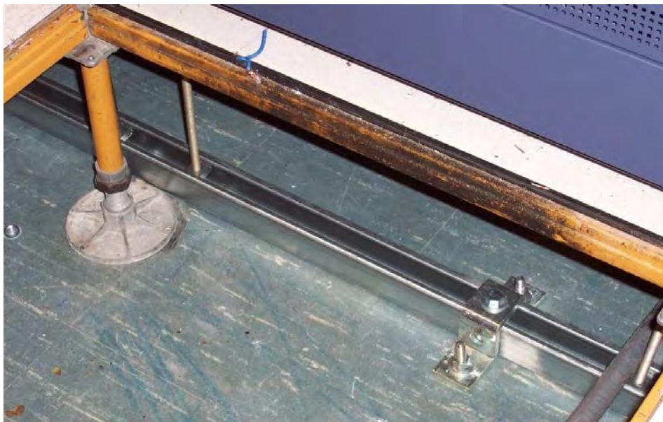
Figure 14-20 Illustration of Securing Cabinets and Racks on an Access Floor to a Concrete Slab Using Threaded Rod and Steel Channel
